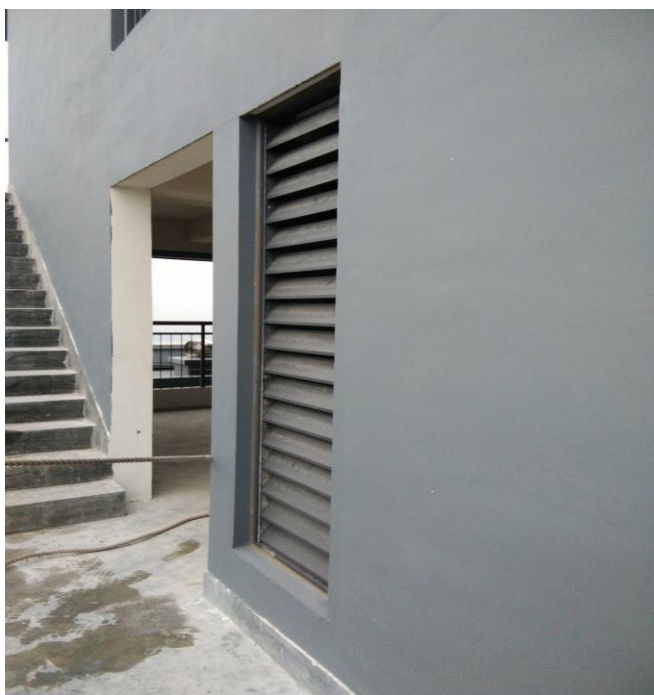
12-2#楼楼顶发电机排烟井窗
